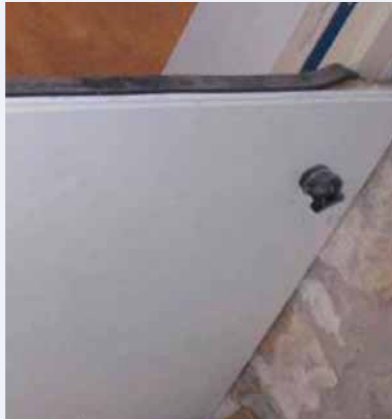
Figure 3 Door guard fitted to the internal door way
